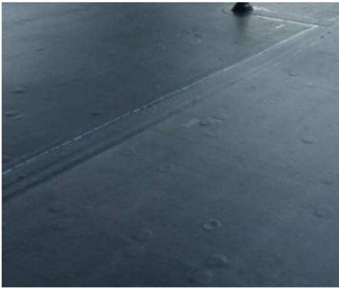
BLACK EPDM (SLOPED GARAGE ROOF)
