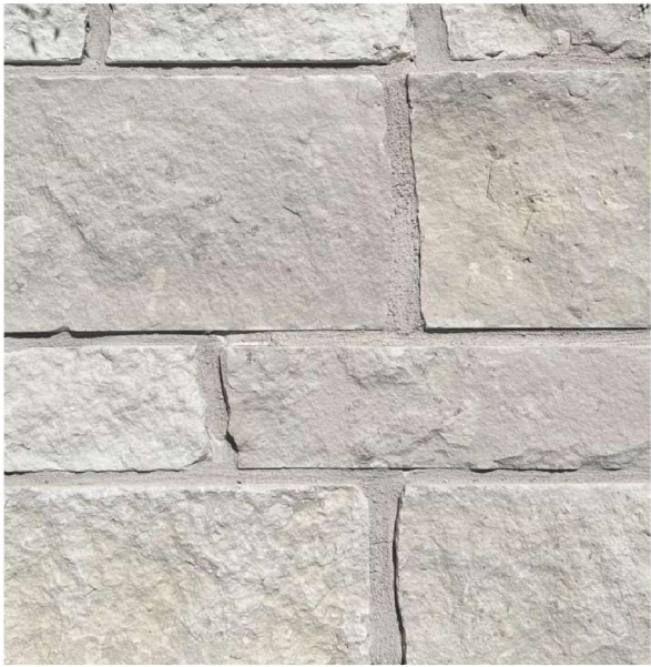
LYRA LIMESTONE MOCKUP PRIOR TO INSTALL
